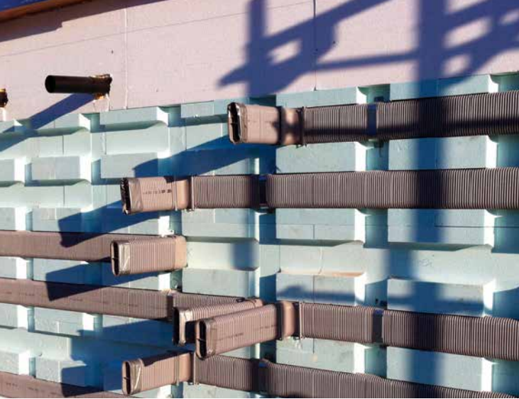
Multifunctional facade elements with insulation panels (EPS) and integrated ducts made of polymer pipes. © Fraunhofer ISE
