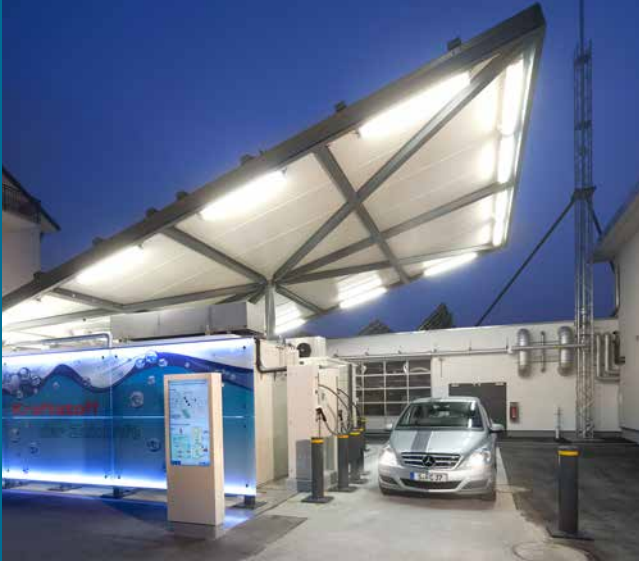
Solare Wasserstoff-Tankstelle am Fraunhofer ISE in Freiburg. © Fraunhofer ISE
